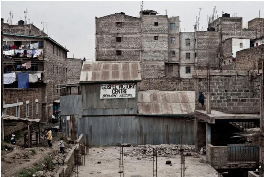
One of the oldest “slum” neighborhoods of Nairobi, Mathare is a sprawling and crowded metropolis with densely packed housing, unpaved streets and buildings constructed in exposed concrete block and sheets of tin. Francesco Giusti
